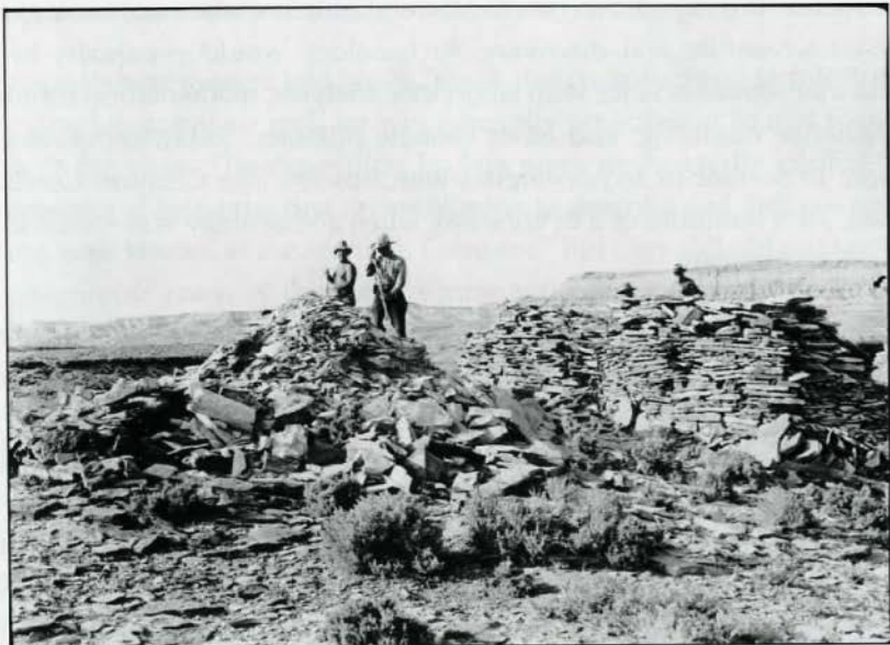
The Clafin-Emerson crew excavating in Lower Hill Creek (ET6-26) on July 29, 1931.
