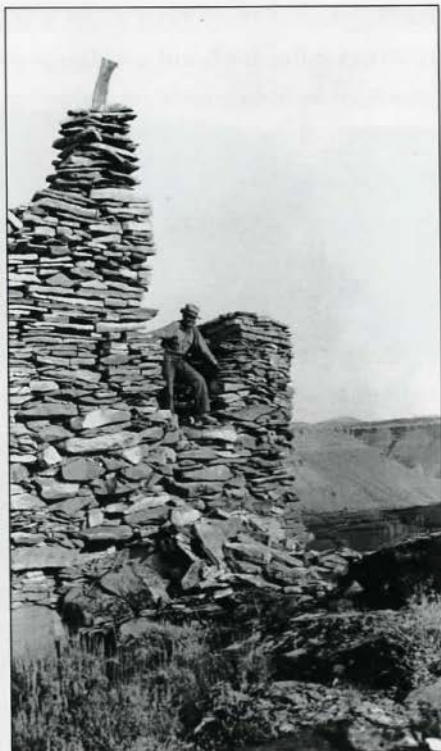
A massive stone tower at Fort Rocking Chair (ET6-13) above the Taylor Ranch, as photographed on July 27, 1931.
